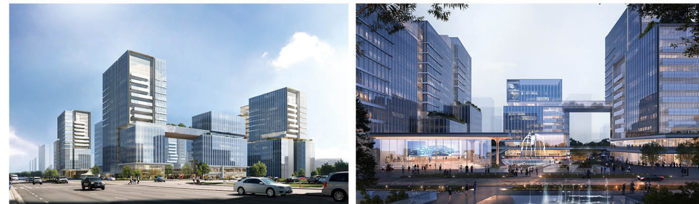
Curtain Wall Project of Taizhou Digital Science and Technology Park
